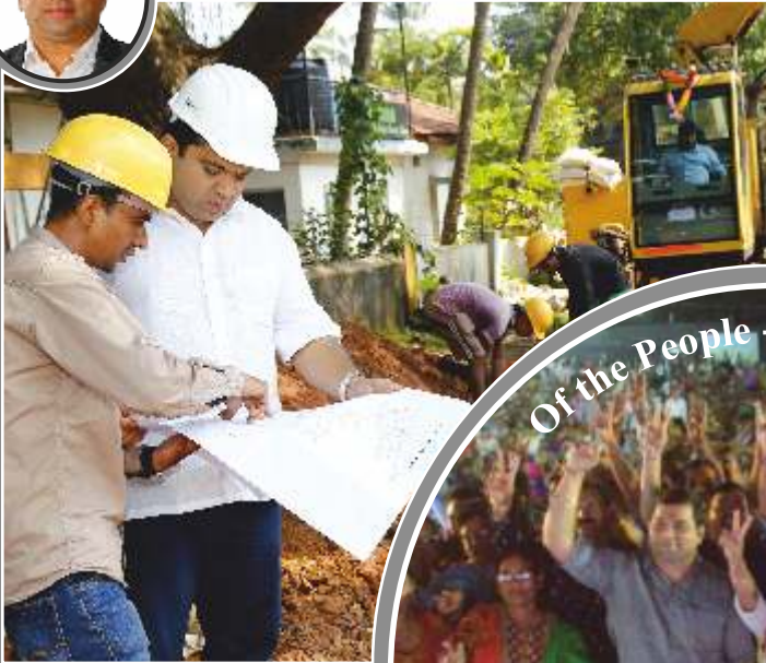
Sewerage pipeline laid for a healthier Tomorrow
